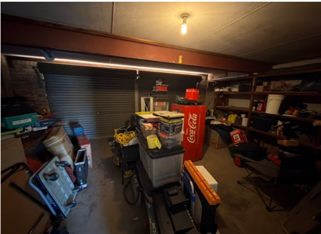
The garage area is in serviceable condition.
