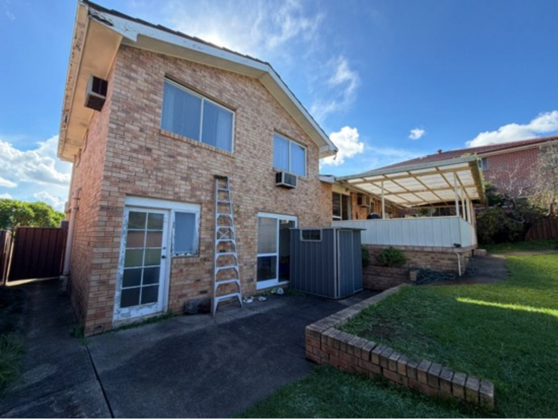
Exterior windows and doors present in serviceable condition for the age.
