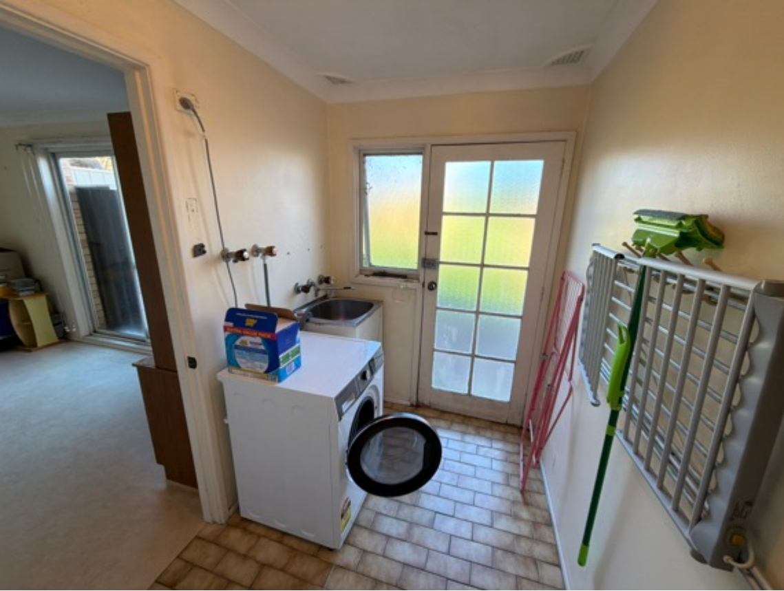
The laundry is in serviceable condition.
