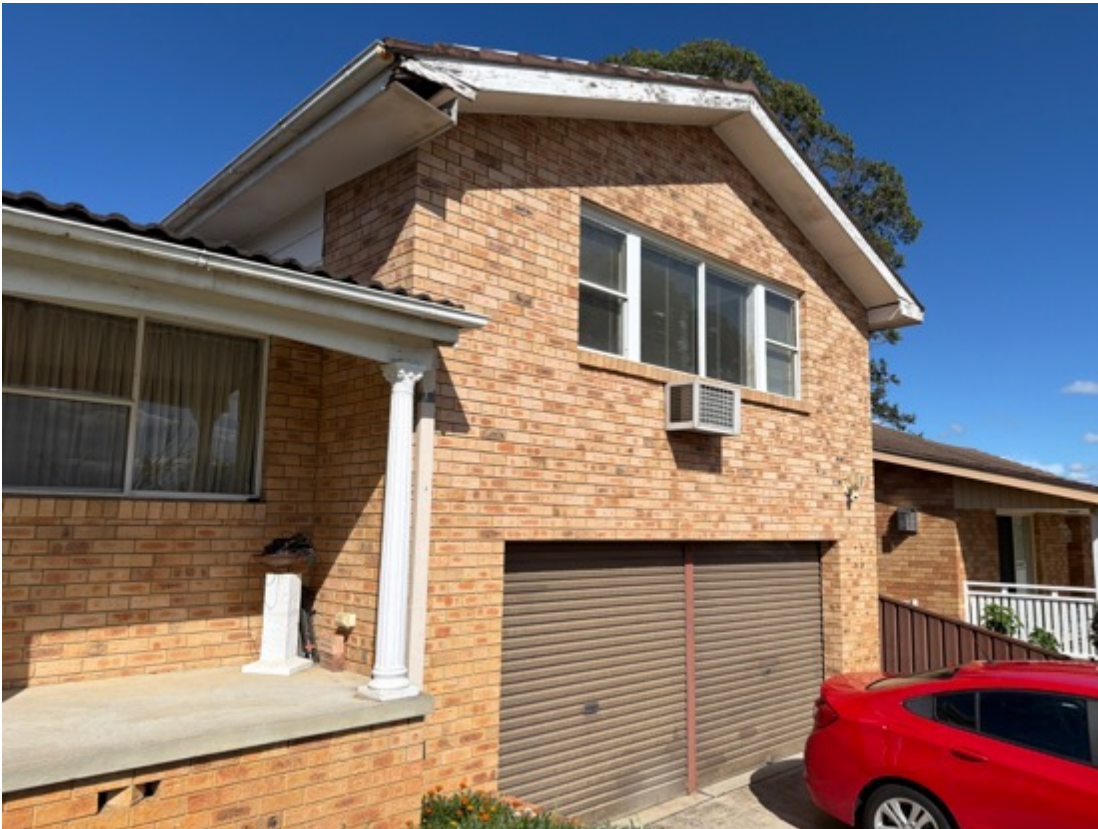
Garage roller doors tested, functioned at the time of inspection (manual function, surfaces display low level blemishes.)
