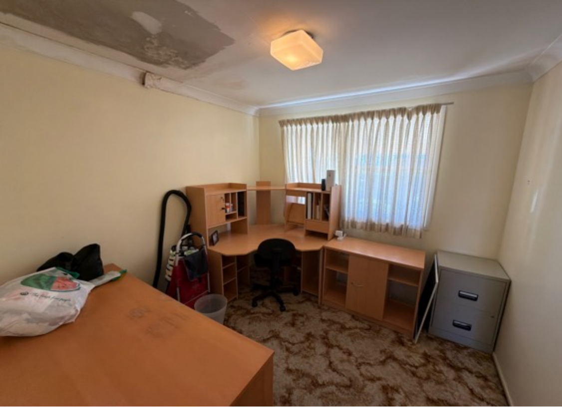
Interior bedroom areas present in serviceable condition for the age - renovations are required due to the age.
