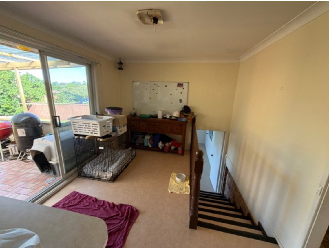
Steel internal lights require checking by a licensed electrician.
