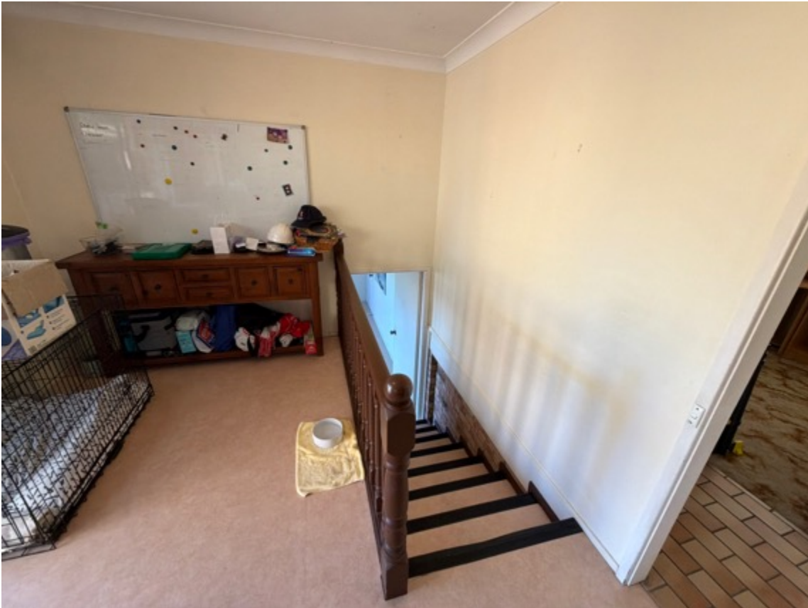
Interior railings checked are structurally sound.
