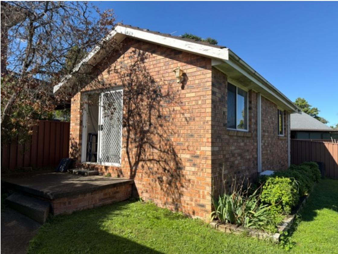
The rear granny flat is in serviceable condition, renovations are required due to the age.
