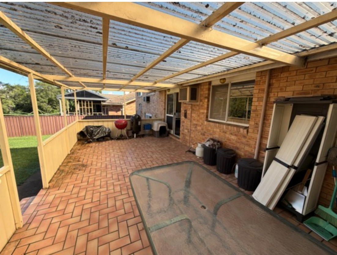
The rear pergola checked is structurally sound.
